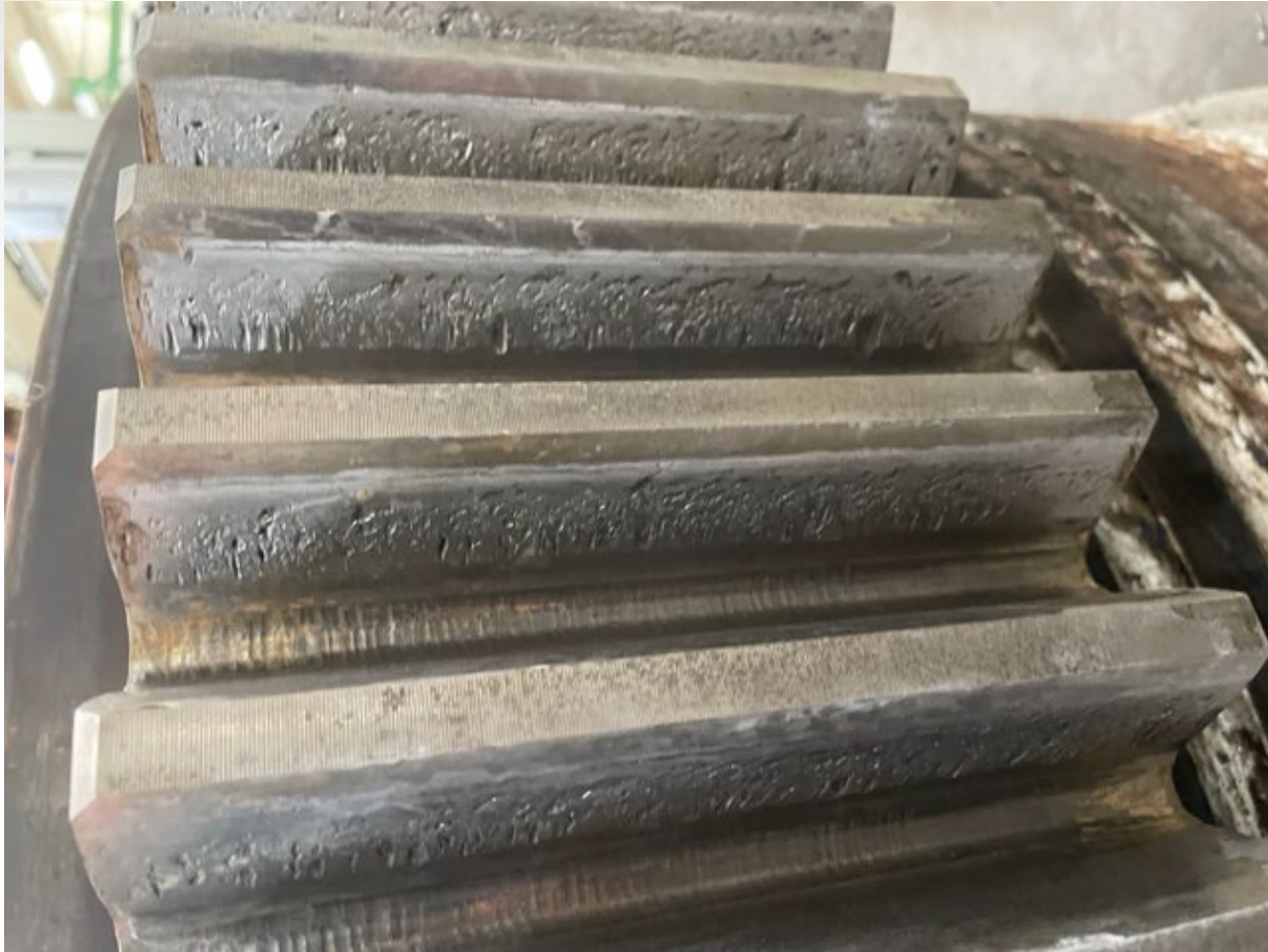
Pitted north drum gear
